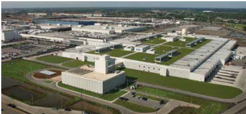
Siplast Teranap was installed on this automobile manufacturing facility in Michigan, creating the world's largest green roof.
