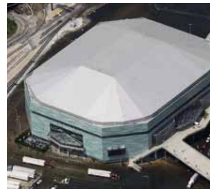
▲ Siplast aluminum Veral, installed in 1998, protects the New Orleans Sports Arena.
