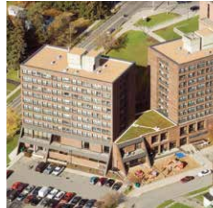
▲ Siplast NVS Lightweight Insulating Concrete and Paradiene 20/30 were chosen for the dormitories on this university in New York. The dormitories are connected by a corridor that features a Teranap Green Roof System.
