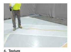
Immediately broadcast Pro Texture Beads into the wet embed-ment layer of Pro Color Finish Resin before it sets using a hopper gun. Backroll to fully embed the Pro Texture Beads into the wet resin.
