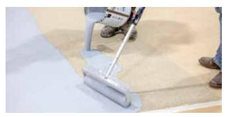
3. Color Coat Install a layer of Pro Color Finish using a roller over the Pro Natural Quartz.
