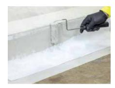
2. Over the primed substrate, apply a base coat of catalyzed Terapro Flashing Resin at with a roller or brush. Work Pro Fleece reinforcement into the wet, catalyzed flashing resin base coat using a roller or brush to fully embed the fleece in the resin and remove trapped air.
