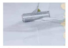
3. Embedment Layer Install a layer of Pro Color Finish using a roller.
