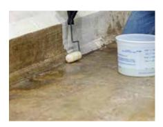
Using tape, mask the perimeter of the area to be flashed to ensure a clean edge. Prime the substrate with Pro Primer W or Pro Primer T (depending on substrate) and allow to cure for 45 minutes.
