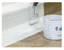
Apply an even top coat of Terapro Flashing Resin immediately following embedment of the fleece to ensure full saturation of the fleece. Remove tape before the resin sets.
