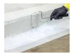
Over the primed substrate, apply a base coat of catalyzed Terapro Flashing Resin at with a roller or brush. Work Pro Fleece reinforcement into the wet, catalyzed flashing resin base coat using a roller or brush to fully embed the fleece in the resin and remove trapped air.
