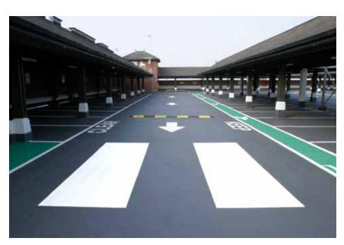
The finished application is ready for vehicular traffic after 3 hours..
