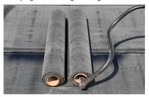
5. After back-rolling, fully torch the Teranap-series finish ply to the Paradiene 20 TG-series base ply in one direction. Concentrate the heat where the Teranap finish ply and the Paradiene 20 TG-series plies make contact. Torch uniformly, side-to-side, using an "L" motion to preheat the selvage of the previous sheet. Lap sides and ends a minimum of 4 inches.
