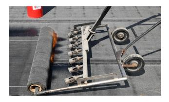
4. Alternatively, the roll can be unrolled in its entirety, set into place, and rolled back from each end to the center of the roll. Using this technique assists in keeping the roll straight during installation.
