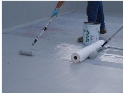
5. Apply a top coat of catalyzed Parapro Roof Membrane Resin using a roller immediately following embedment of the Pro Fleece to ensure full saturation of the fleece. Allow to cure for 2 hours prior to application of any optional color finishes or anti-skid surfacings. The completed Parapro Roof Membrane can be exposed to foot traffic after a 2-hour cure time.
