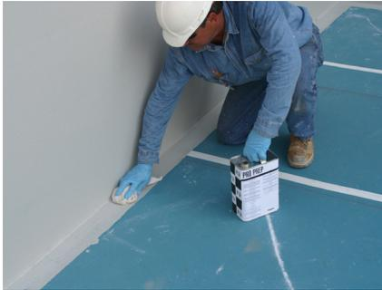
1. Using Pro Prep, wipe down thoroughly all horizontal areas of the Parapro Flashing Membrane which will receive an overlap of the Parapro Roof Membrane. Allow Pro Prep a minimum 20 minutes drying time before continuing.
