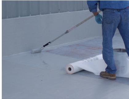
2. Note that certain substrates require priming with Pro Primer before application of Parapro Roof Membrane Resin. Refer to the Substrate Preparation Chart for priming requirements. Apply a base coat of catalyzed Parapro Roof Membrane Resin using an approved stub roller.
