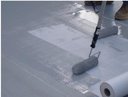
4. Use a roller to embed the fleece and remove trapped air. Lap fleece layers a minimum of 2 inches, and apply an additional coat of catalyzed Parapro Roof Membrane Resin between layers of overlapping fleece.
