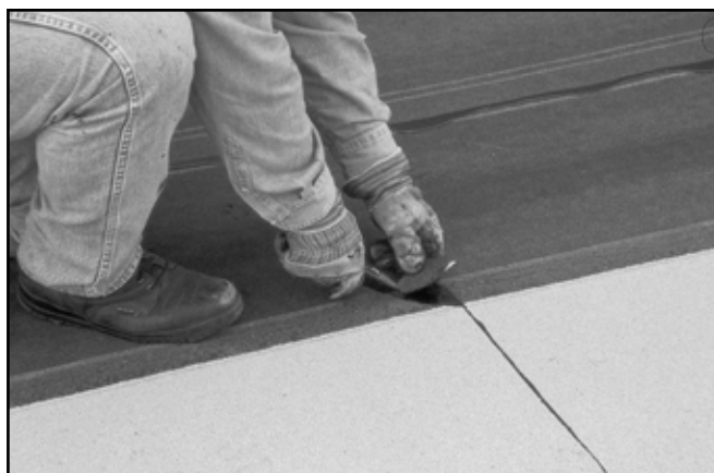
At end laps, make a "dog ear" angle cut on the overlapping selvage edge.
