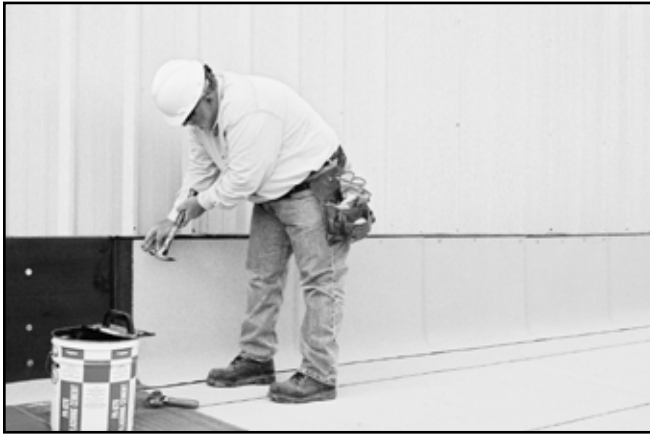
Mechanically fasten the top edge of the Paradiene 40 FR flashing sheet.
