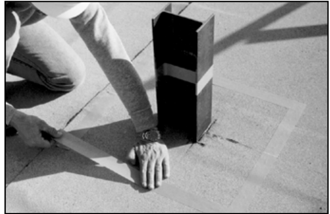
Using masking tape, mask off the area to be covered with Parapro 123 Flashing. Mask the termination of the flashing 6 inches high on the I-beam, and extending 8 inches onto the finished roof membrane in all directions. Catalyzed Parapro Flashing Resin must extend ¼-inch beyond Pro Fleece. Masking tape should be placed accordingly.
