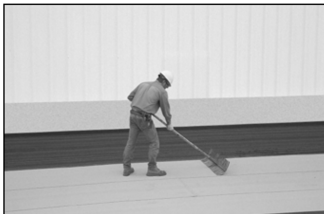
Apply pressure on the sheet to ensure full contact with the substrate and complete embedment in the adhesive. Heat welding the laps is recommended with certain applications and weather conditions.
