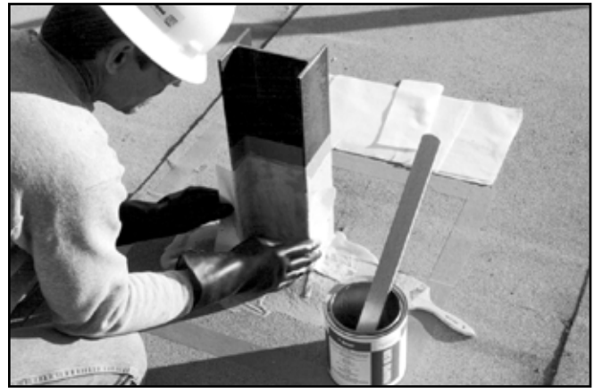
Apply catalyzed Parapro Flashing Resin to the vertical surfaces, at a minimum consumption rate of 0.19 kg/sf (2.0 kg/m 2 ), extending onto the finished membrane a minimum of 2 inches. Apply the pre-cut Pro Fleece to the vertical surfaces, and embed the fleece in catalyzed resin, extending the resin ¼-inch beyond the edge of the fleece. Ensure that no air pockets are trapped beneath the fleece. Saturate all fleece surfaces with catalyzed Parapro Flashing Resin prior to overlapping with additional fleece. Strips of fleece must overlap by at least 2 inches.
