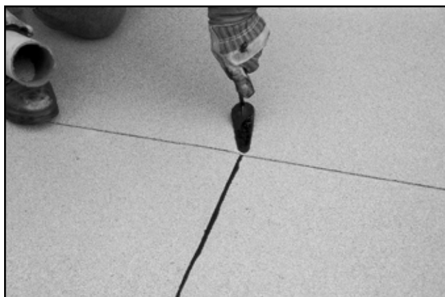
Using a clean trowel, apply pressure to top seal all edges at T-laps.
