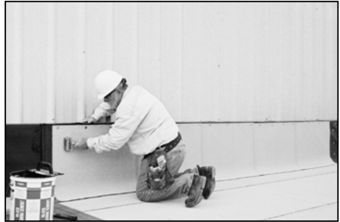
Using a roller, apply pressure to the surface of the Paradiene 40 FR flashing sheet to ensure complete contact with the substrate.
