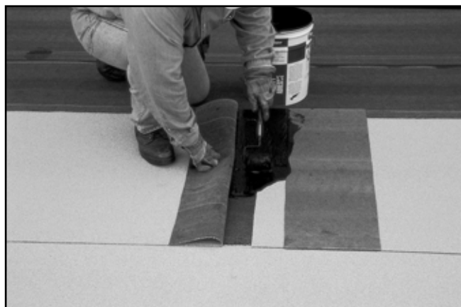
Use a slop sheet at end lap locations to allow for a full application of PA-311 Adhesive under the sheet and provide a neat finished appearance. On granule-surfaced materials, end lap usage of PA-311 adhesive should be approximately double that of the field sheet.
