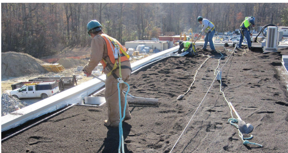
Fine grading of ParaGREEN Growing Media with rake
