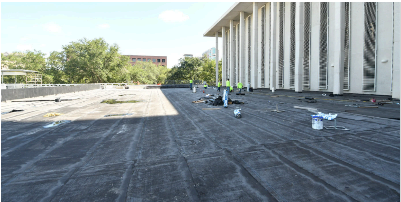
Completed Teranap SBS membrane assembly prior to installation of the overburden.
