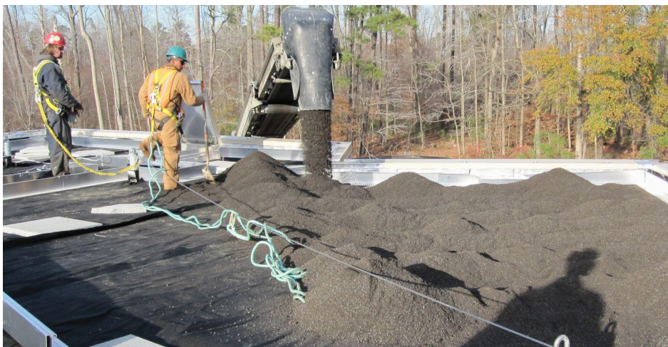
ParaGREEN Growing Media installed utilizing a conveyor
