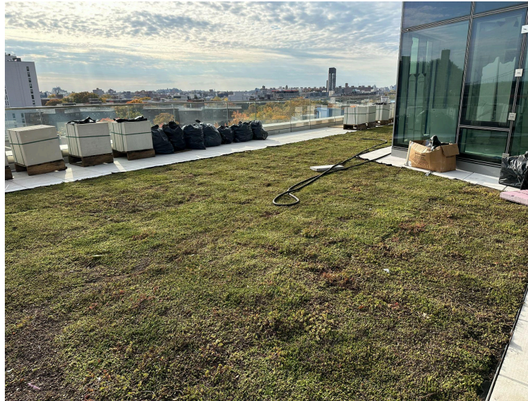
Completed ParaGREEN Sedum Mat installation.
