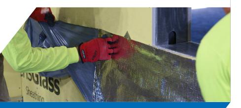
WALLcontrol™ Reinforced Aluminum AWB and Flashings feature a temperature-stable butyl adhesive and reinforced aluminum topsheet, engineered for enhanced performance in wall assembly areas exposed to elevated temperatures.
