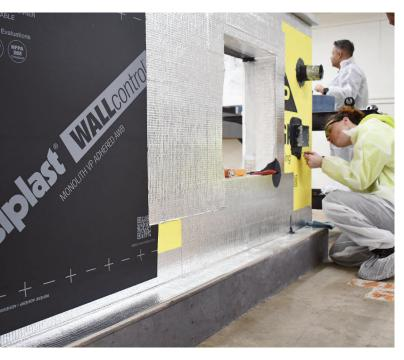
WALLcontrol Reinforced Aluminum Butyl-Adhered AWB is a primerless, self-adhered, non-vapor-permeable, UV-resistant AWB designed for any time of the year with its high-temperature stability and low-temperature application. This solution is durable and flexible, serving as both an air-barrier membrane and a water-resistive barrier for commercial wall systems.
