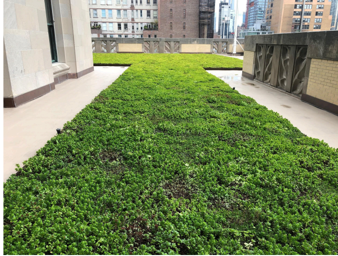
Figure 4: A vegetated roof installed over a conventional roof system with a reflective membrane.
