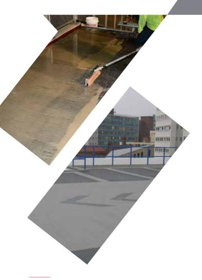
The Terapro VTS Pro Grid Reinforced system provides an efficient application with the same hard-wearing surfacing as our traditional Pro Fleece Reinforced system.
