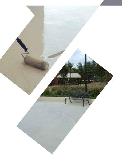
The fast-curing chemistry and resilient physical properties of the Terapro unreinforced PMMA system make it a great choice for those unoccupied spaces that require a fast return to service.
