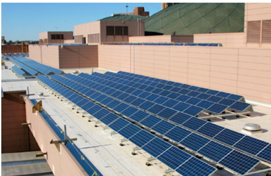
This photo is showing a large solar array that is mechanically attached to the structure at the corners and the quarter points along the leading edge.
