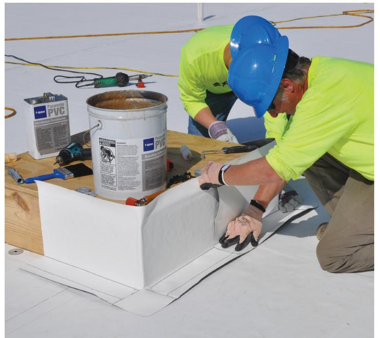
Prefabricated Parasolo PVC, KEE and TPX accessories are an efficient way to address detail conditions.
