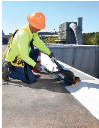
Apply a patch of Paradiene 20 TG to extend 3 inches in all directions from the damage/puncture.
