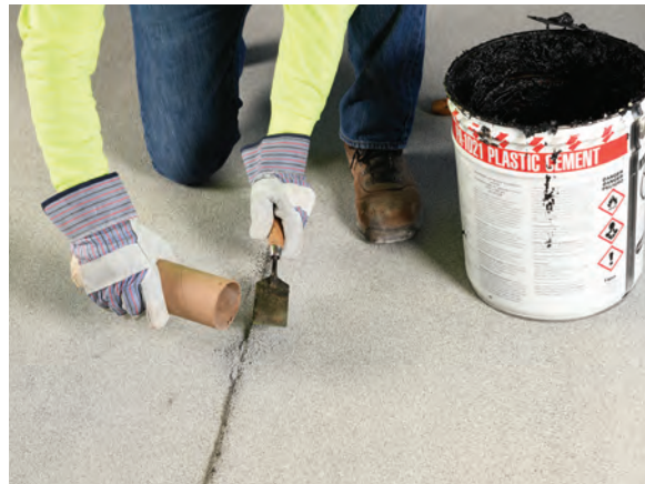
Use a clean trowel or roller to press the lap down and ensure full adhesion. Apply granules over bleed-out.
