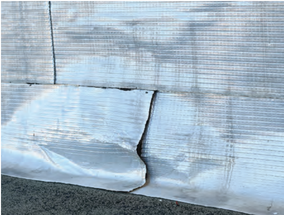
Blister in the Veral flashing membrane.
