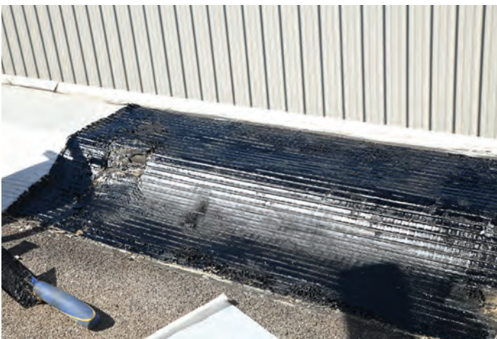
Using a torch, carefully heat and remove the foil surfacing to expose the underlying bituminous membrane to receive the repair patch.
