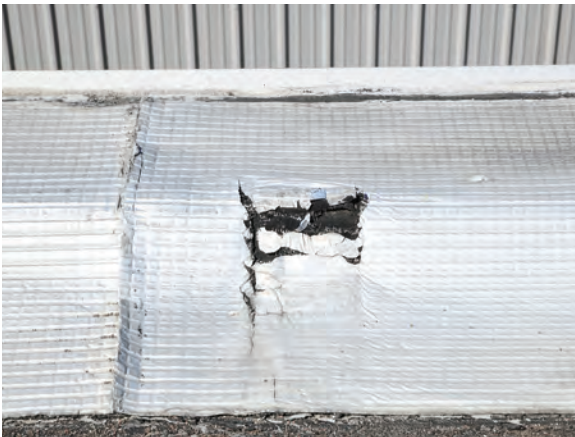
Damaged/punctured Veral flashing membrane.
