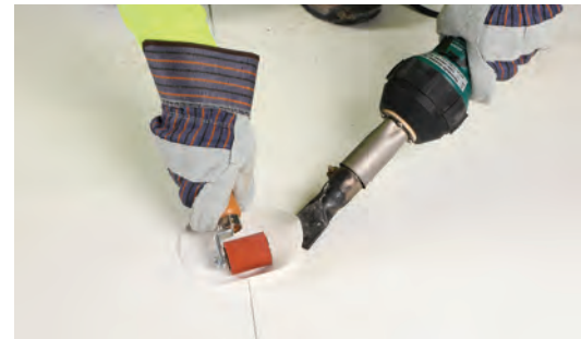
Use a hand-held hot air welder with an appropriate fitting to resealed the loose membrane lap.
