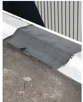
Apply a patch of Paradiene 20 TG to extend 3 inches in all directions from the damage/puncture.
