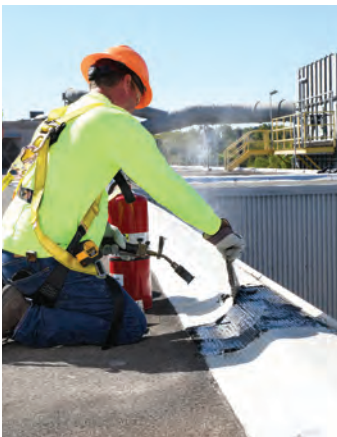
Using a torch, carefully heat and remove the foil surfacing to expose the underlying bituminous membrane to receive the repair patch.
