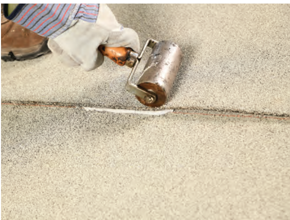
Use a clean trowel or roller to press the lap down and ensure full adhesion.
