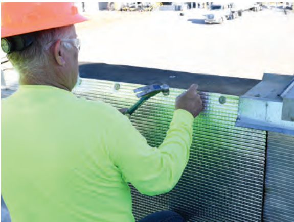
Fasten the top of the new flashing piece on 9-inch centers.
