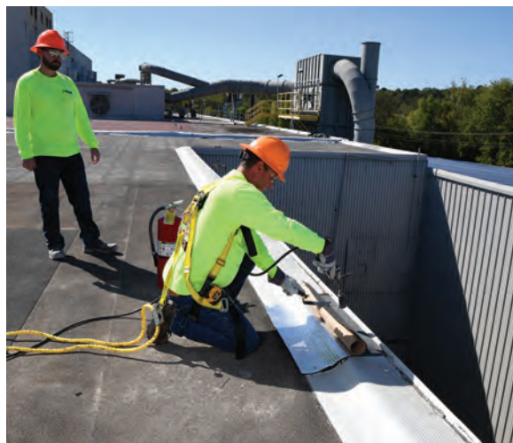
Apply the new flashing membrane to extend from lap to lap.
