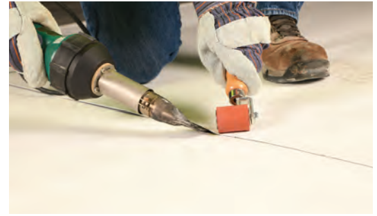
Use a hand-held hot air welder with an appropriate fitting to resealed the loose membrane lap.
