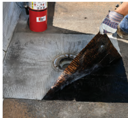
Remove the strainer, clamping ring and delaminate any aluminum foil surfacing from the drain sump flashing (if applicable).
