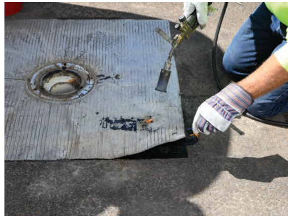
Remove the strainer, clamping ring and delaminate any aluminum foil surfacing from the drain sump flashing (if applicable).
