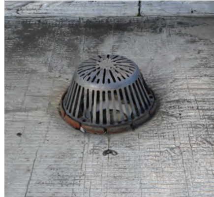
Roof drain flashing in need of reworking.
