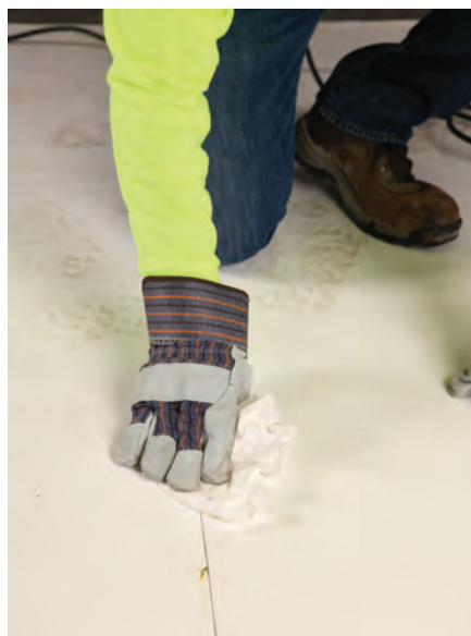
Dirt stains can be removed using an all purpose household cleaner. The membrane must also be prepared by cleaning wiping with Parasolo Membrane Conditioner.
