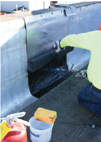
Fasten the top of the new flashing piece on 9-inch centers.
