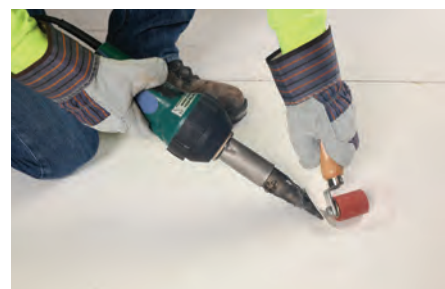
Small punctures can often be patched with pre-cut Parasolo PVC Patches.
