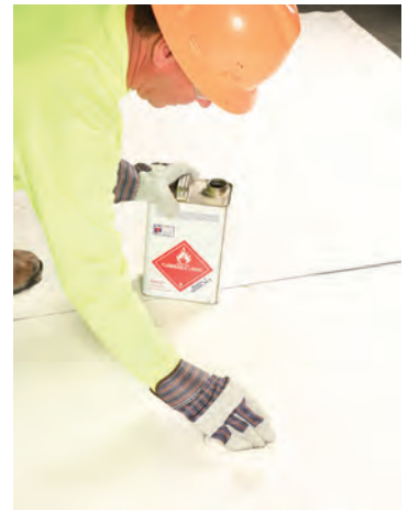
Dirt stains can be removed using an all purpose household cleaner. The membrane must also be prepared by cleaning wiping with Parasolo Membrane Conditioner.
