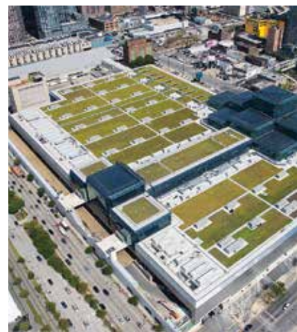
New York's Jacob K. Javits Convention Center features a 5,000-square green roof assembly that includes Siplast NVS Lightweight Insulating Concrete, Paradiene 20 HV TG, Teranap, pavers, and Paraguard Coping.
