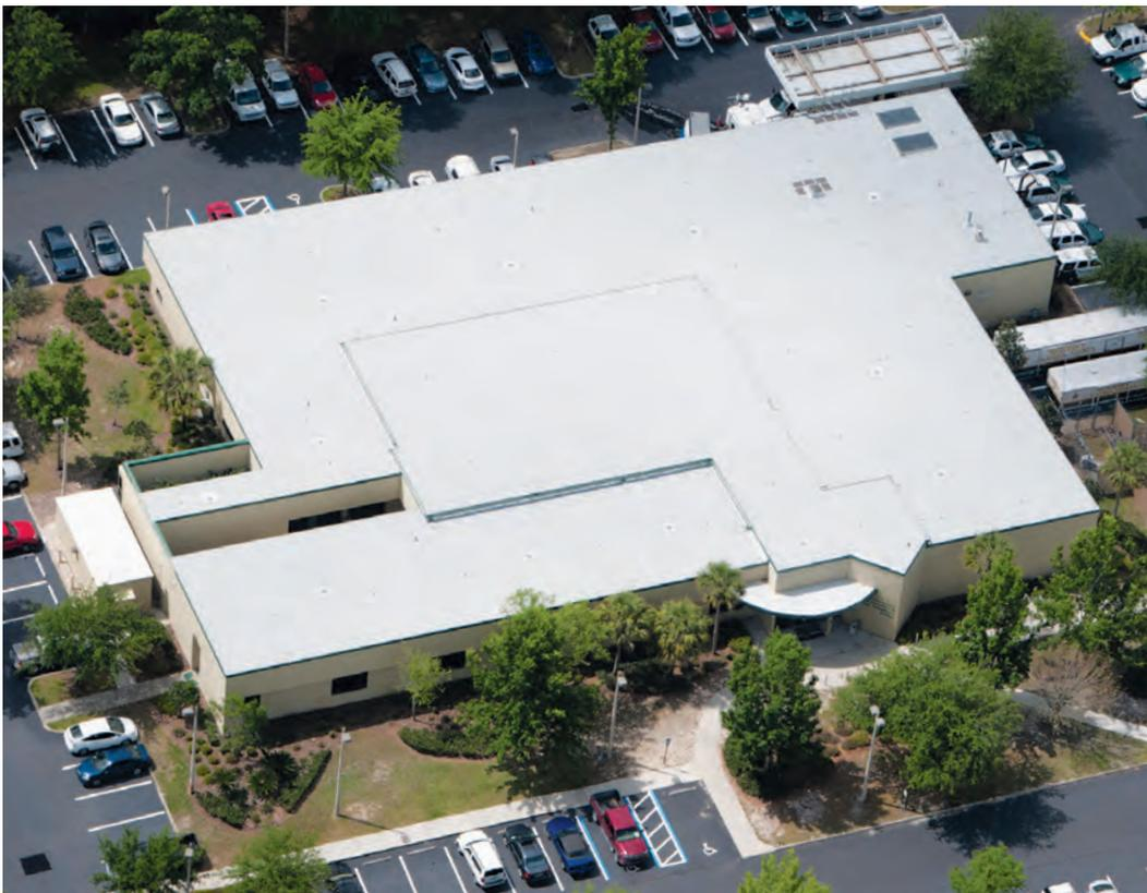
To meet the high performance needs of the critical Alachua County 911 Center, the time-proven, two-ply Siplast SBS-modified bitumen Paradiene 20/30 Eco-Activ® System was chosen. In addition, reusable Siplast NVS Lightweight Insulating Concrete roof insulation was installed on the project.
