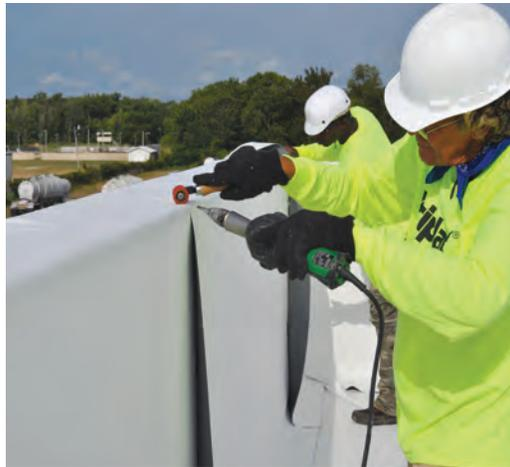
Parasolo PVC KEE brings the Siplast service level and commitment to projects appropriate for single-ply applications. Consistent heat welding and rolling seams helps ensure a successful application.
