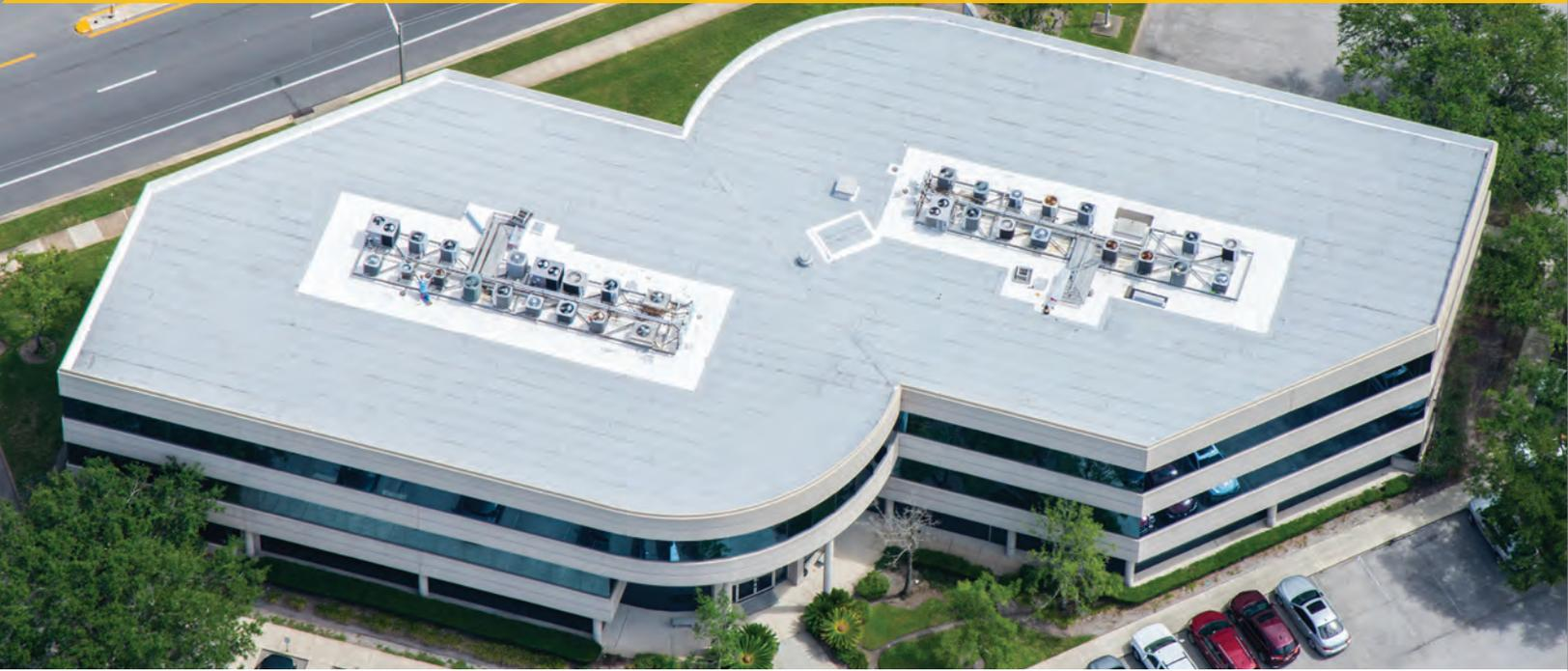
Parapro Roof Membrane provides an excellent solution for the area surrounding the air handlers on this Paradiene 20 TG/ 30 FR TG roof.
