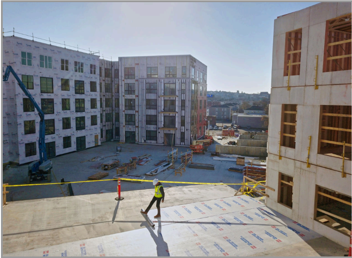
Figure 4: A self-adhering vapor retarder application over a concrete roof deck with a CSP of 3
