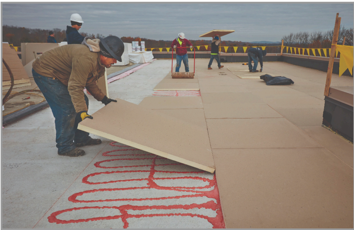
Figure 3: Low-rise foam application over a concrete roof deck with a CSP of 2
