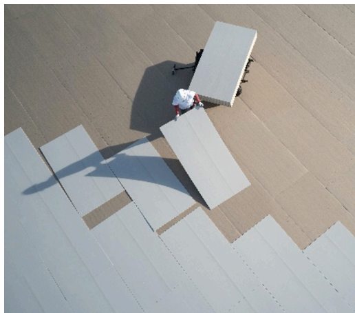
Image 2. HD polyiso cover board installation. Image courtesy of GAF.
