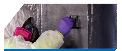
WALLcontrol Liquid AWB is applicable by roller and sprayer to enable ease of installation in projects with complex wall assemblies, rough surfaces, or numerous penetrations.
