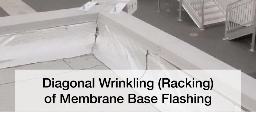
Diagonal wrinkles in membrane base flashing, commonly referred to as "racking," sometimes occur along the parapet walls. This condition can affect the long-term performance of a roof membrane system. The wrinkles manifest above the cant strip and extend along vertical surfaces of the wall area. Such wrinkles are more frequent at wall areas near the corners of the building.
