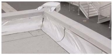
Siplast Veral - Aluminum-clad SBS-modified Bitumen
